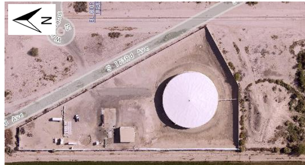
Aerial view of the existing facility.
