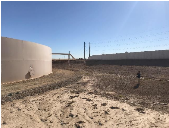
South of the existing tank- looking east.
