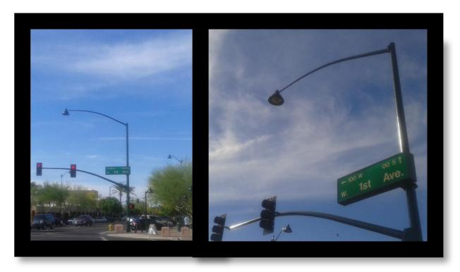
Note: In this photo, the ADOT style traffic signal structure has a decorative lighting fixture added to the street light and has been powder coated green to add to the aesthetics of this district.
