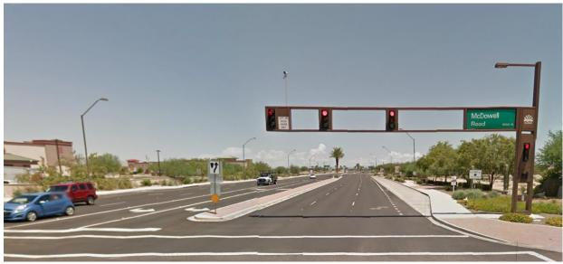
Note: An ADOT mast arm can be fabricated 15 feet longer than a Modular Traffic Signal, providing for the red arrow to be over the left turn lanes.
