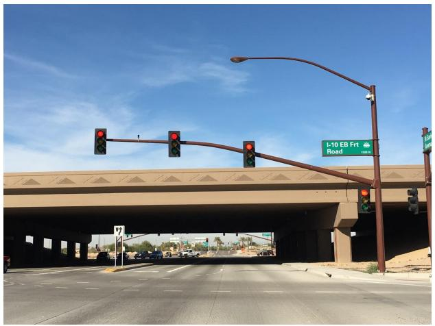
Note: The ADOT style traffic signal structure has been enhanced with powder coated brown to match Goodyear's existing traffic signal structures.
