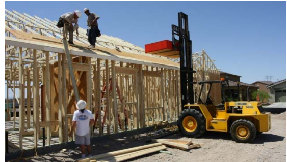
Figure 5.6 Construction of a new home
