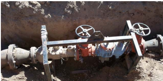
Figure 5.5 Waterline replacement
