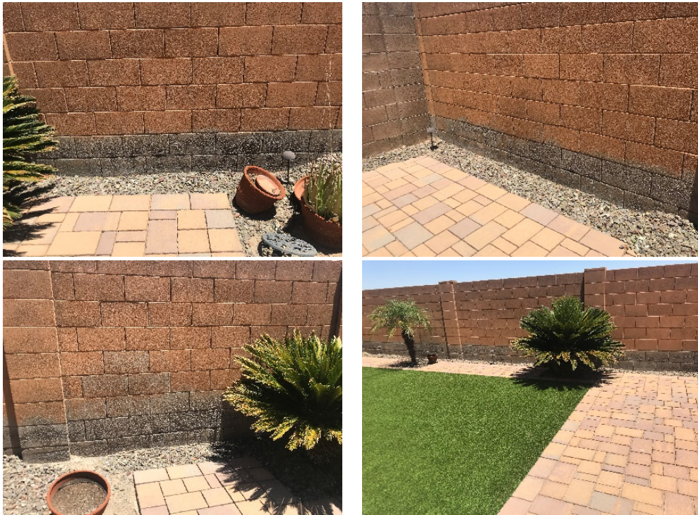
Figure 15. House No. 271 Wall Inspection
