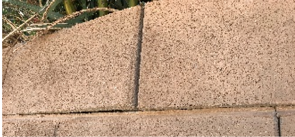
Figure 11. Examples of Bulging Blocks
